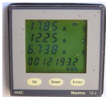
Photograph 23 - IME NEMO 72-L power meter
