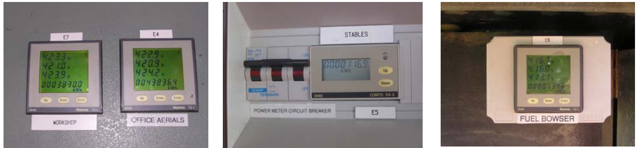
Photograph 34 - Installed power meters E4, E5, E6 and E7 at Feedlot F
