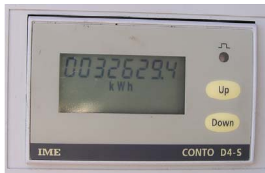
Photograph 24 - IME CONTO D4-S power meter
