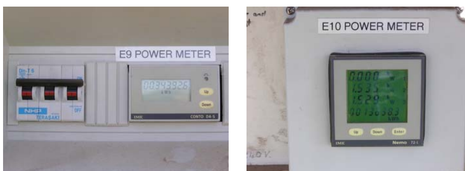
Photograph 29 - Installed power meters E9 and E10 at Feedlot B
