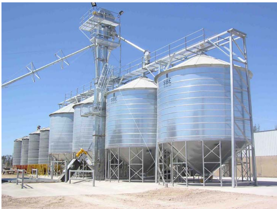
Photograph 1 - Typical grain storage system
