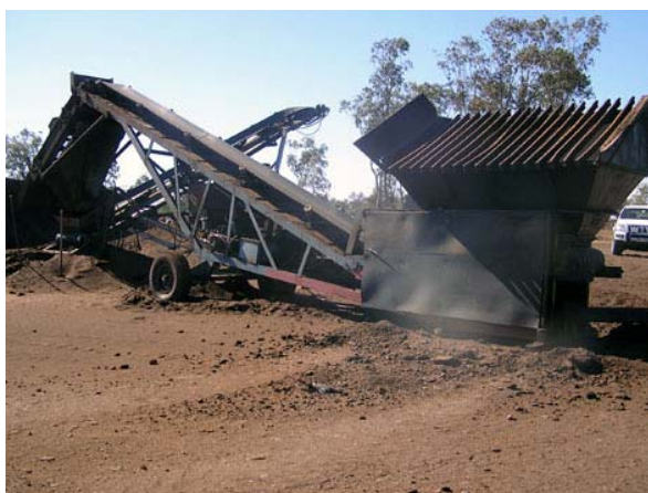
Photograph 18 – Screening machinery at manure stockpile
