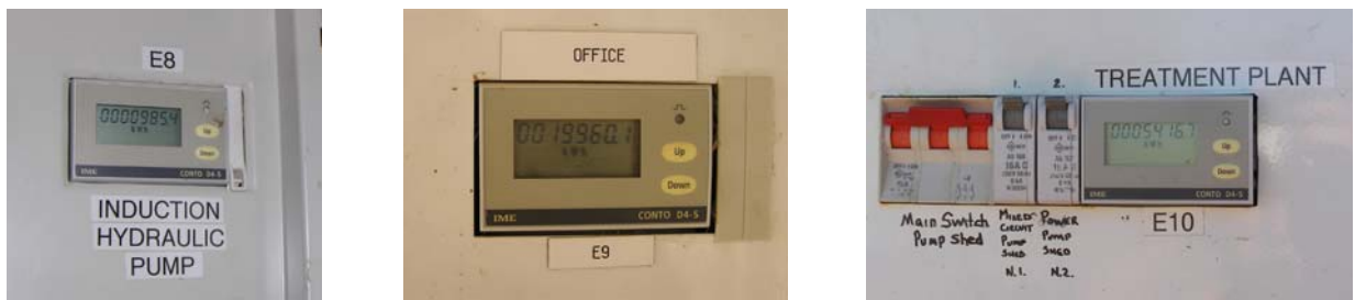
Photograph 35 - Installed power meters E8, E9 and E10 at Feedlot F
