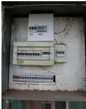
Photograph 26 - Installed power meter E6 at Feedlot A
