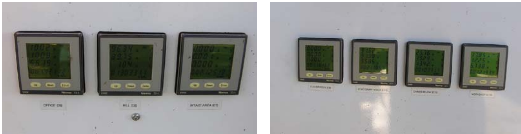
Photograph 30 - Installed power meters E6, E7, E8 (Left) and E9, E10, E15, E16 (Right) at Feedlot D
