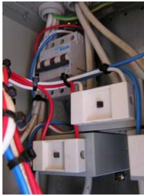
Photograph 25 - Typical installed current transformers
