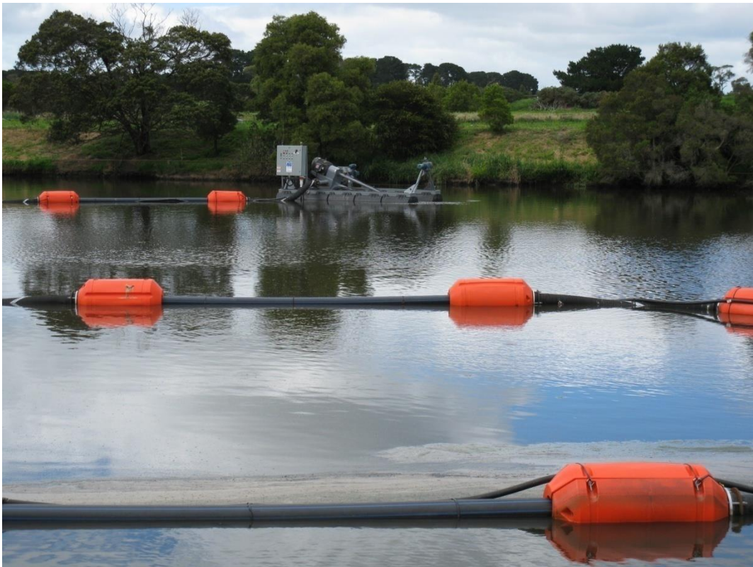
PHOTOGRAPH 12 – POND DREDGE IN OPERATION (DREDGING SOLUTIONS)
