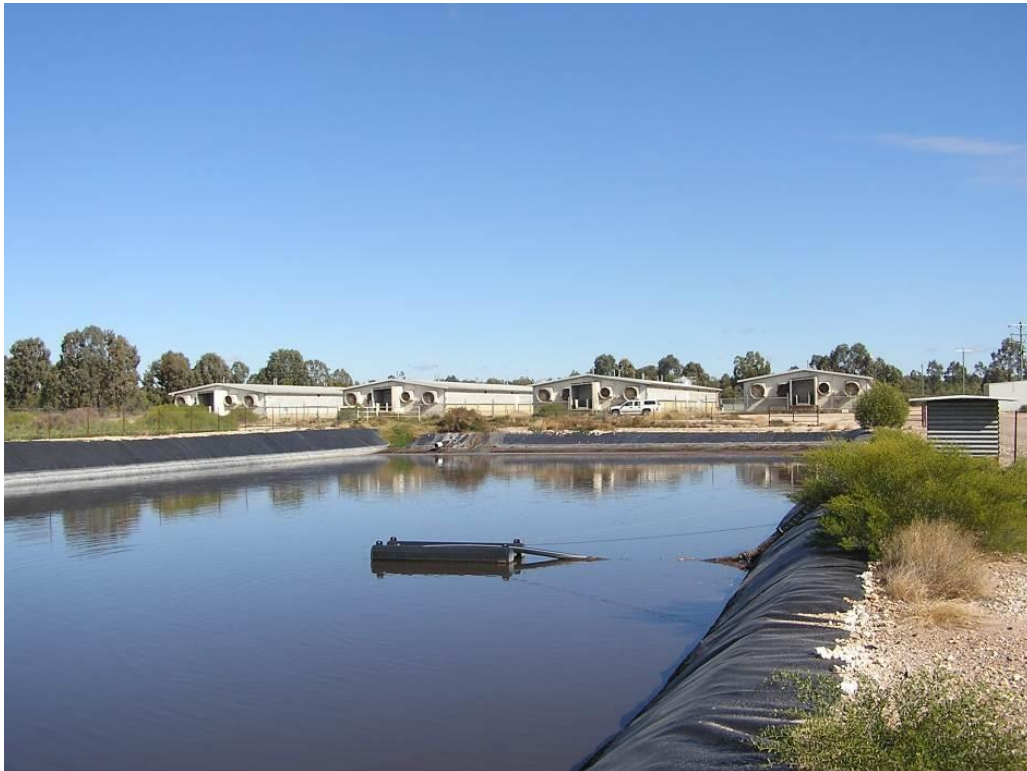
PHOTOGRAPH 30 – PIGGERY D SAMPLING SITE
