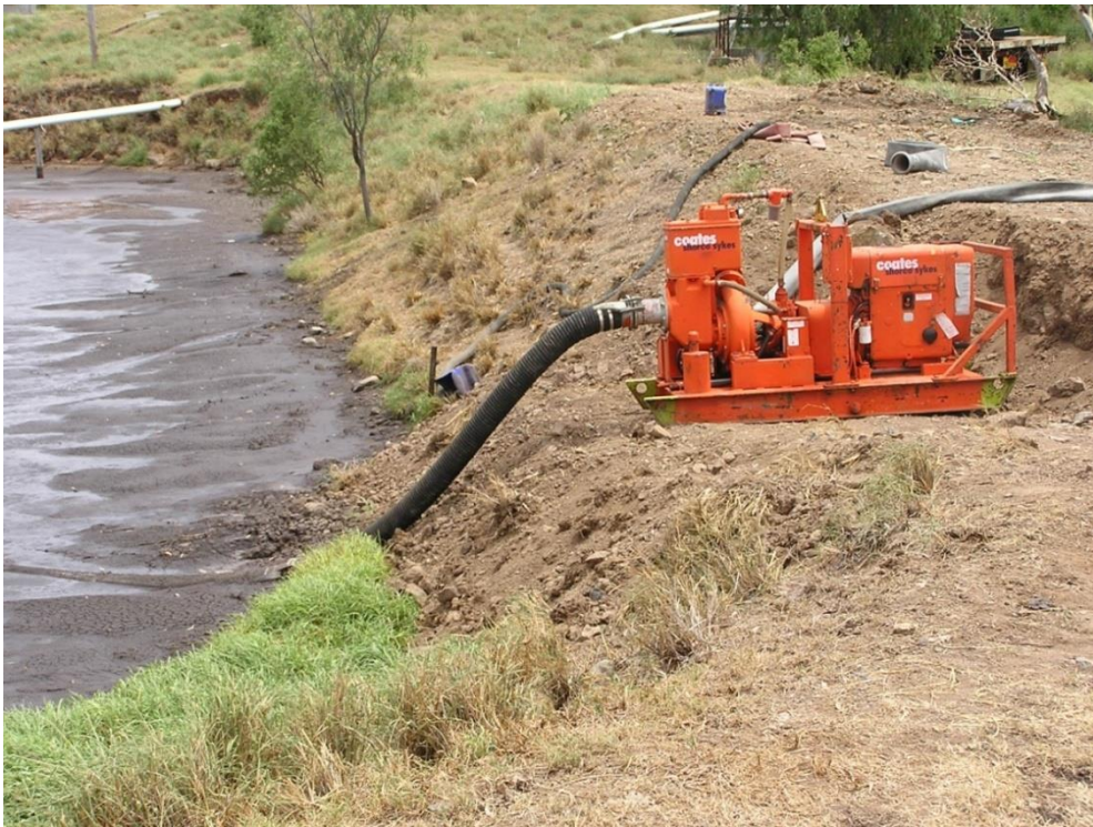
PHOTOGRAPH 5 – DEWATERING AN ANAEROBIC POND PRIOR TO DESLUDGING
