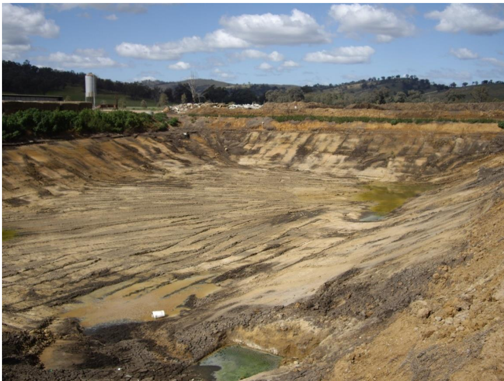
PHOTOGRAPH 8 – ANAEROBIC POND AFTER DEWATERING AND DESLUDGING
