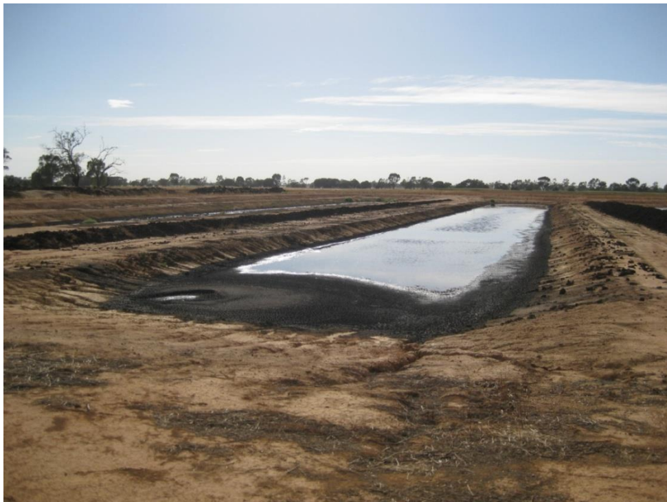
PHOTOGRAPH 21 – NARROW DRYING BAY
