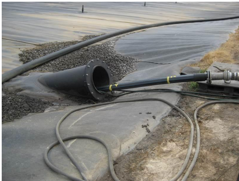
PHOTOGRAPH 40 – SUCTION PIPE INSERTED INTO CAP
