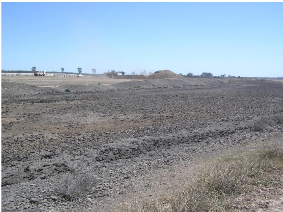
PHOTOGRAPH 6 – DRIED SLUDGE IN A FEEDLOT SEDIMENTATION BASIN READY FOR REMOVAL
