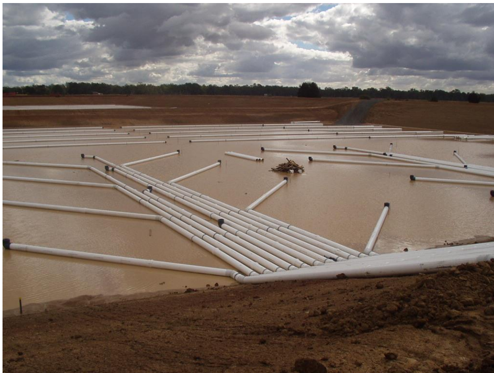
PHOTOGRAPH 15 – INSTALLATION OF SLUDGE REMOVAL PIPE SYSTEM
