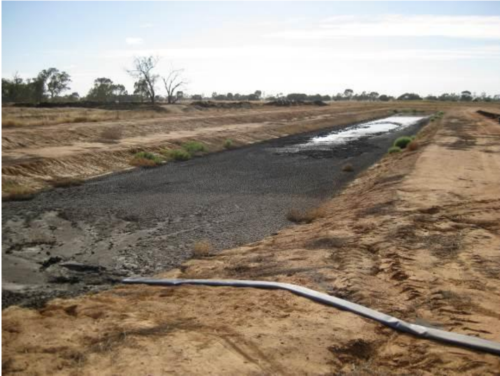
PHOTOGRAPH 27 – PIGGERY A DRYING BAY
