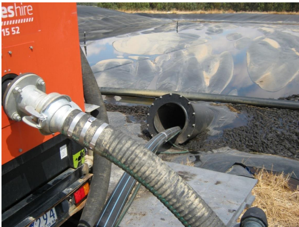
PHOTOGRAPH 17 – PUMP SUCTION PIPE INSERTED INTO IN-SITU DESLUDGING PIPE
