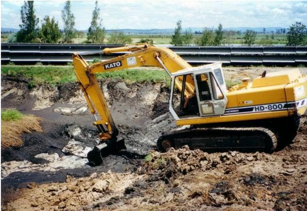
PHOTOGRAPH 7 – SLUDGE REMOVAL FROM A DEWATERED POND WITH AN EXCAVATOR
