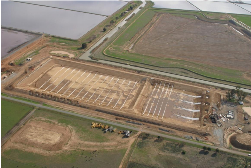
PHOTOGRAPH 14 – INSTALLATION OF SLUDGE REMOVAL PIPE SYSTEM
