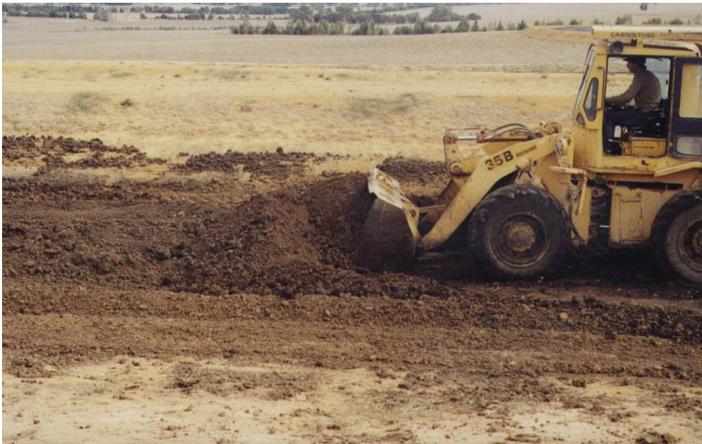
PHOTOGRAPH 24 – SOLIDS REMOVAL FROM DRIED SEPS BAY
