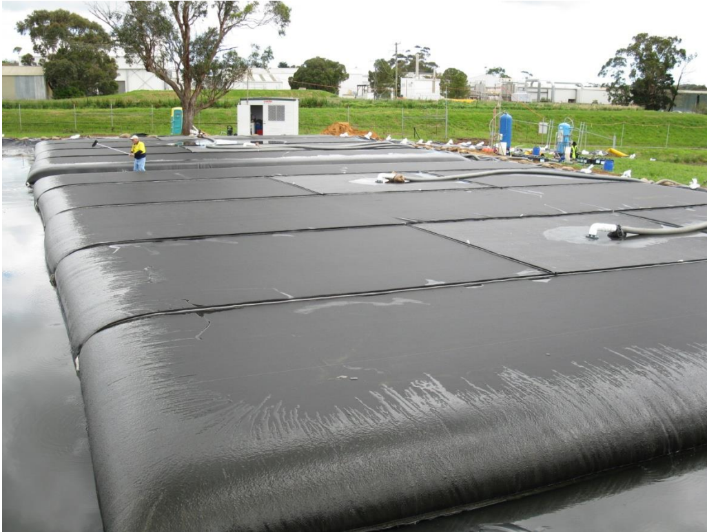
PHOTOGRAPH 26 – DEWATERING SLUDGE USING GEOTEXTILE TUBES (DREDGING SOLUTIONS)
