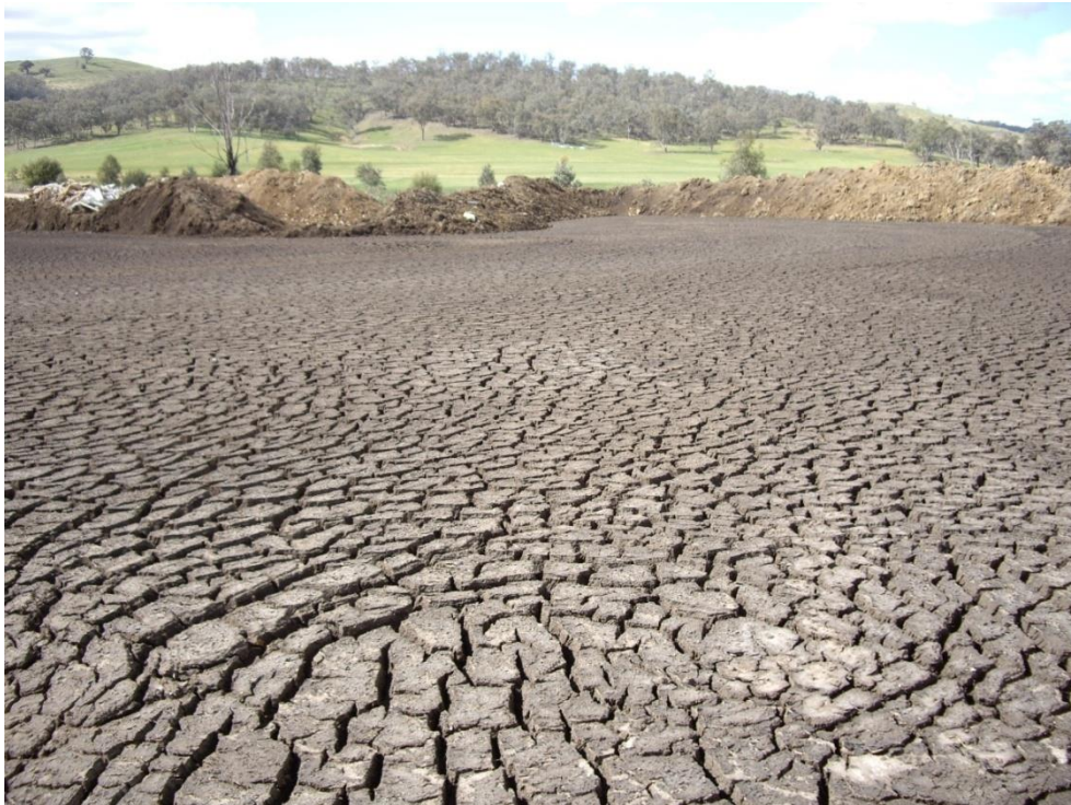
PHOTOGRAPH 20 – SURFACE CRUSTING OF LONG-TERM DRYING BAY
