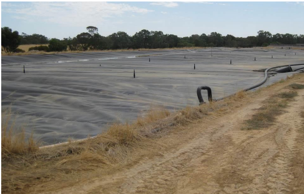
PHOTOGRAPH 1 – COVERED ANAEROBIC POND
