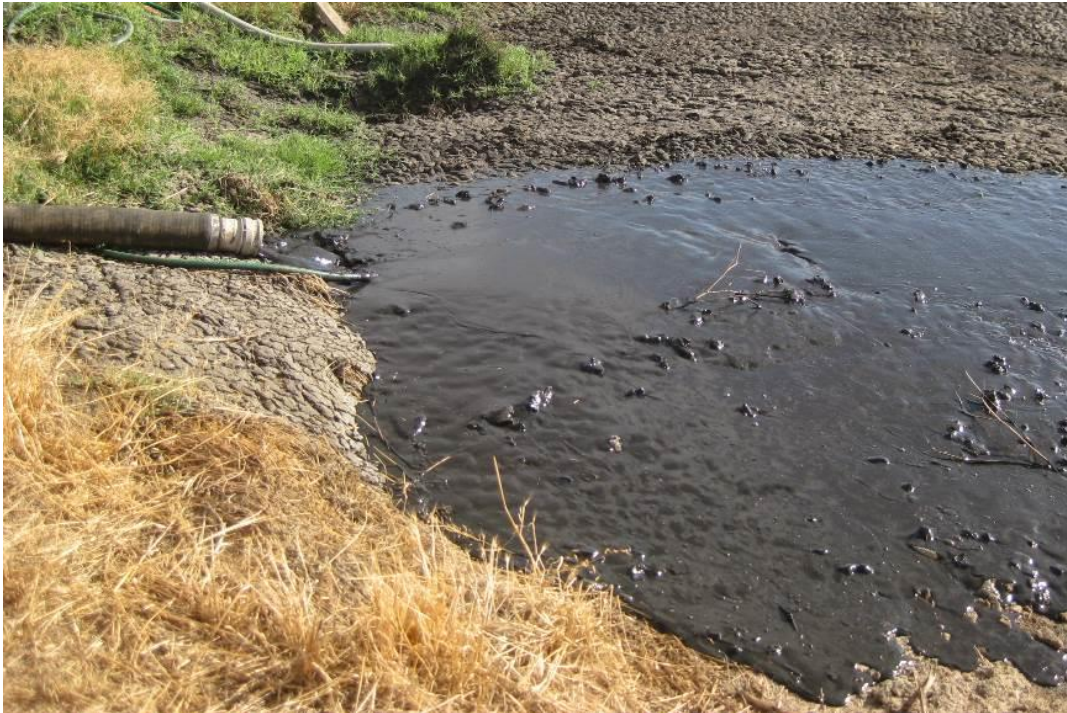
PHOTOGRAPH 44 – SLUDGE REMOVED FROM CAP DURING PUMP PRIMING
