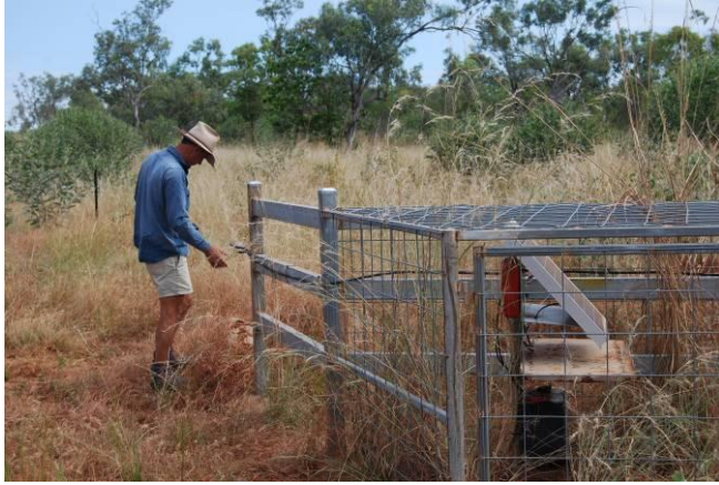
Figure 0.16 Solar panels to power electric fence energisers have proved to be effective on Greenhills.
