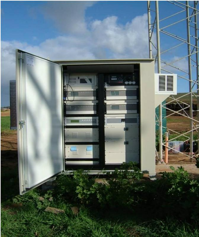
**Plate 6:** Rack-mounted gas analysers in the air-conditioned TGS cabinet.
