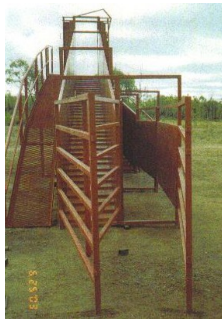
Figure 7. Photographs of double deck loading ramps. The animals are either directed into the right-hand race (which curves inwards to become the lower ramp), or straight ahead to the upper loading ramp. The structure running up the left-hand side of the ramp on the right is a catwalk for stockpersons to assist with loading. These ramps are made by Towers Engineering of Charters Towers in Queensland.
