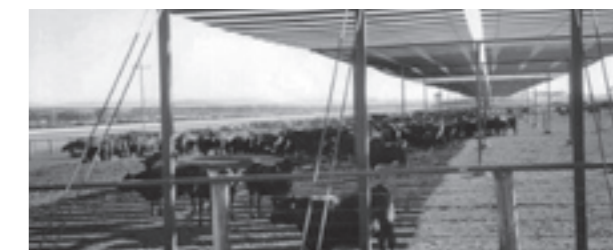
THE MOST EFFECTIVE AND ECONOMIC LEVEL OF SHADE IN FEEDLOTS TO REDUCE HEAT LOAD RISK WAS IDENTIFIED
