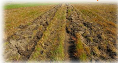
Excess vegetation on mounds
