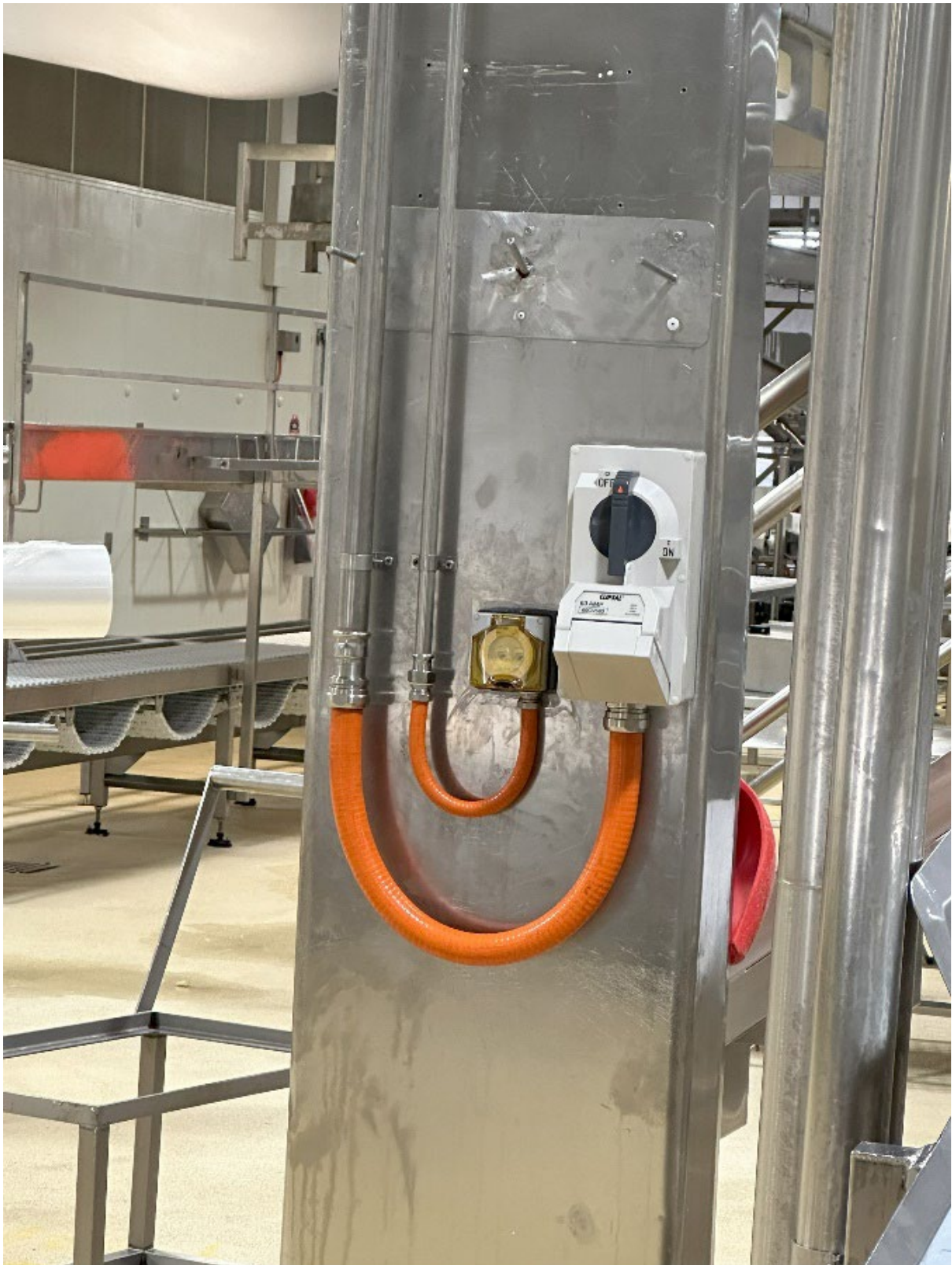
Figure 22 – Room preparation works: Electrical power supply and network connection point.
