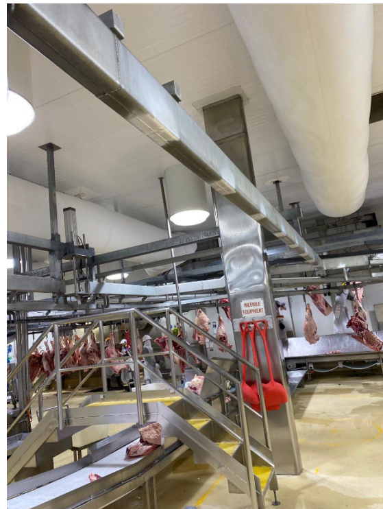
Figure 21 – Room preparation works: Meat rail above robot cell removed & belt conveyor cut back.
