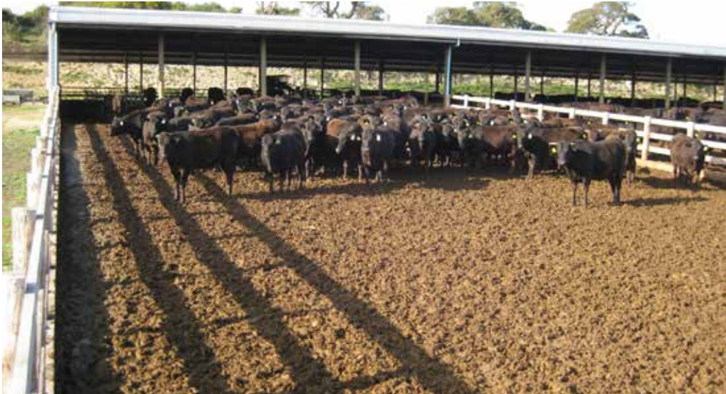
A partially covered (skillion structure) feedlot pen.
