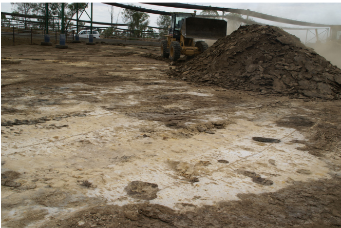
Figure 4: Pen cleaning with a front-end loader where the interface is removed exposing clay base
