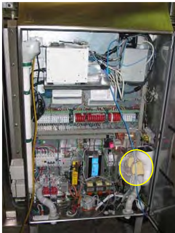
Figure 2-10 Inside slaughter floor control cabinet showing location of safety relays
