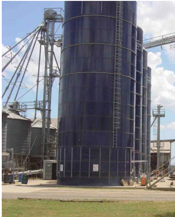
PHOTOGRAPH 7 – TYPICAL RECONSTITUTION SILOS
