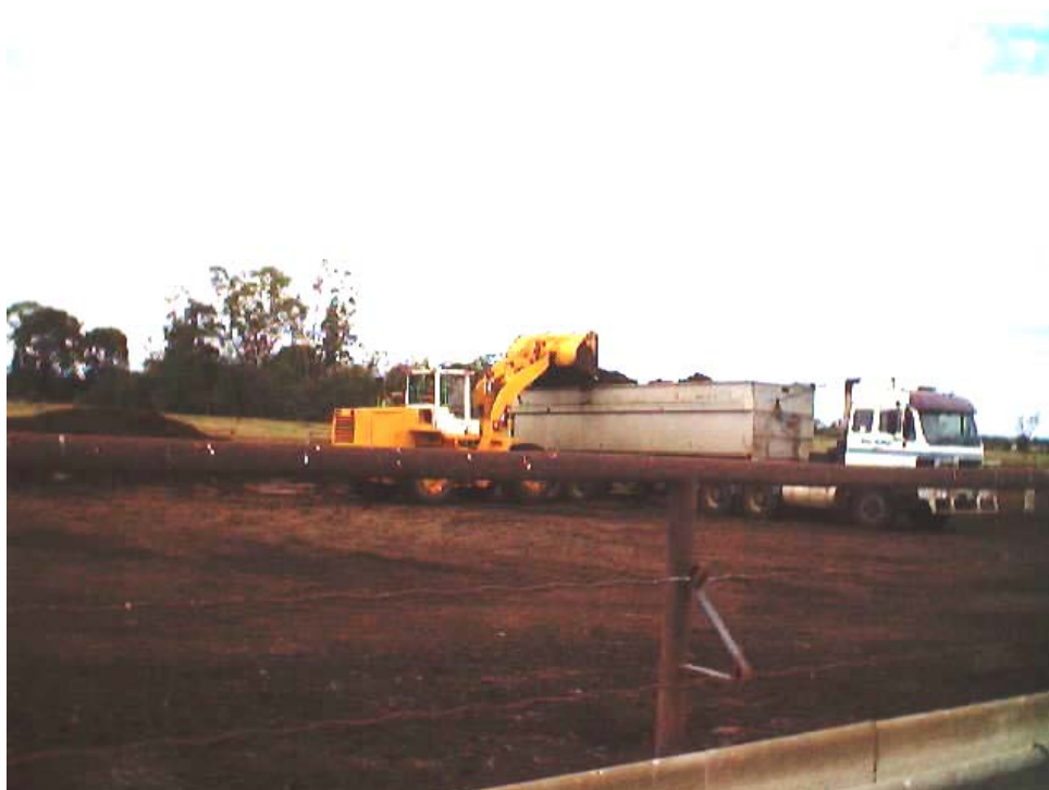
Photograph 3 – Manure removal operation
