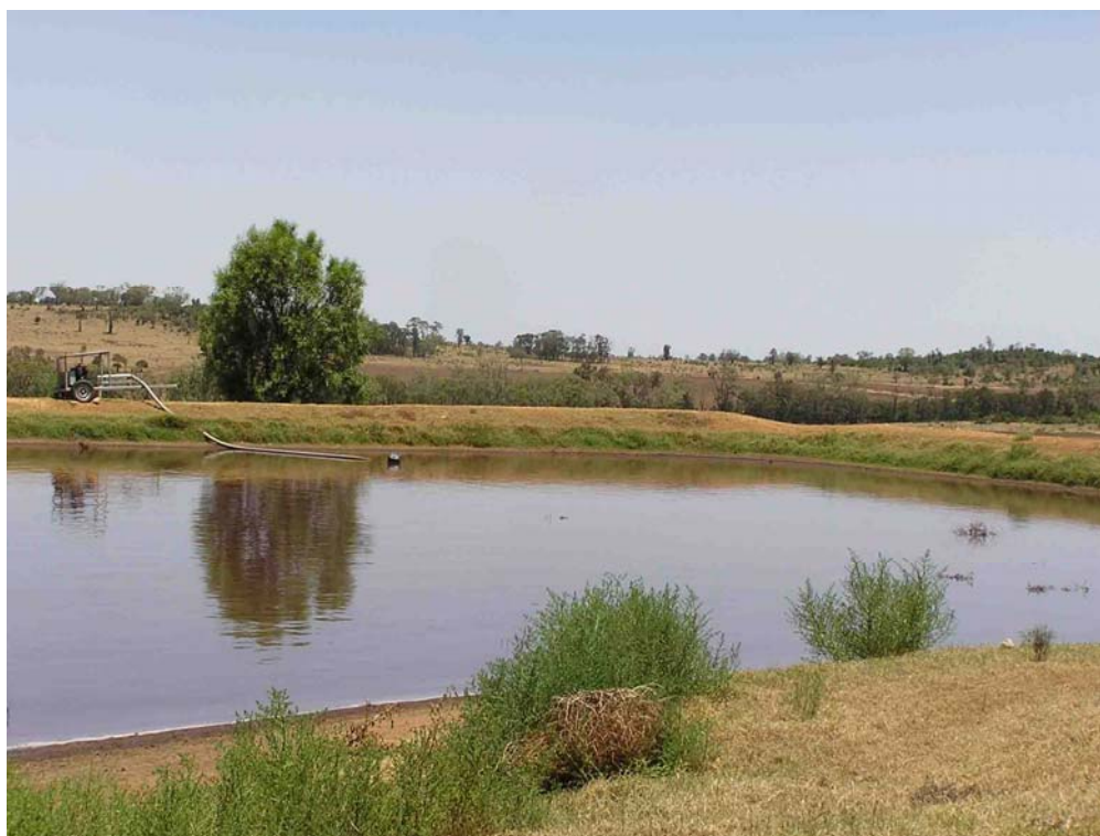
Photograph 11 – Holding pond and associated irrigation pumping equipment
