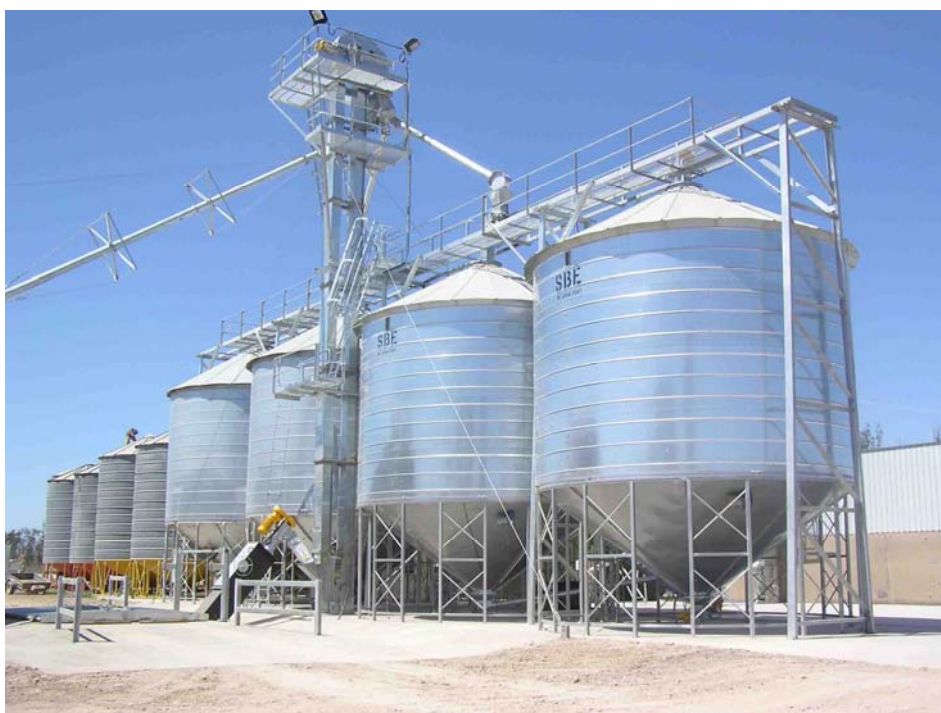
Photograph 4 – Typical grain storage system
