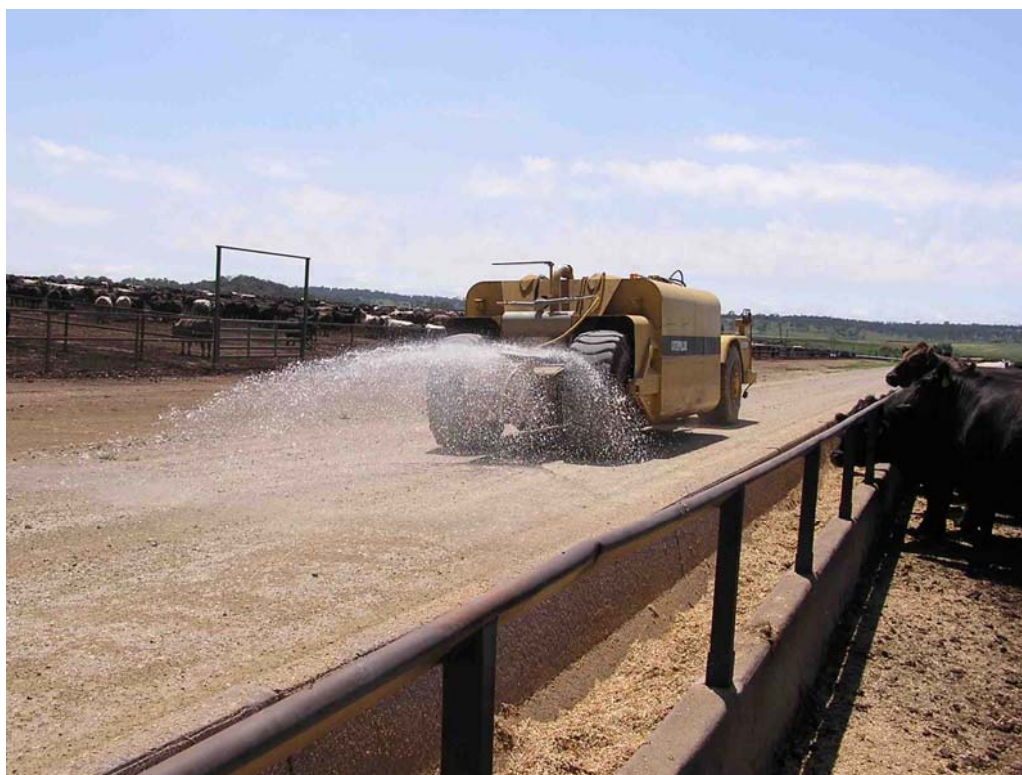
Photograph 6 – Road watering operation
