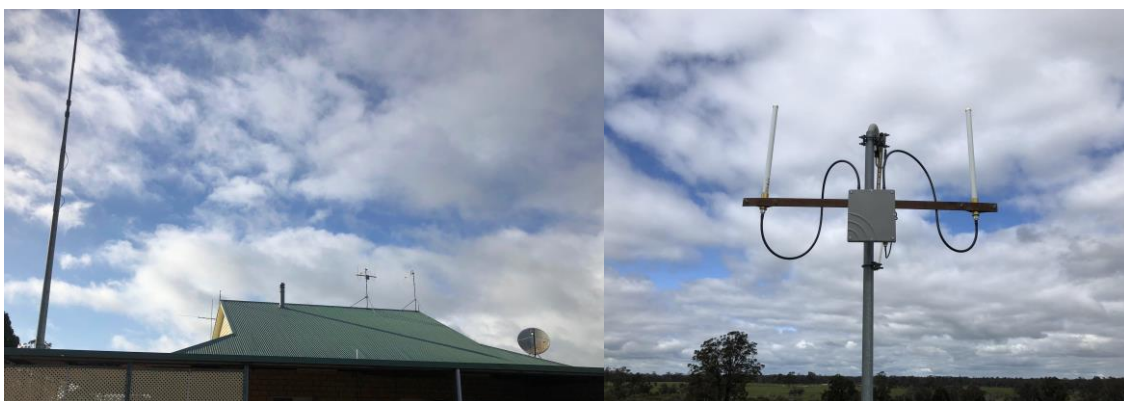
Fig 2: LoRa Gateway install - tag & test
