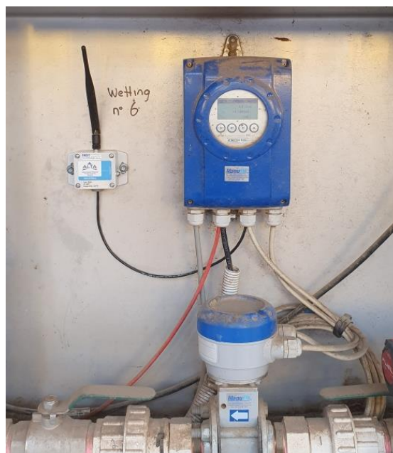
Figure 15: Grain wetting water meter
