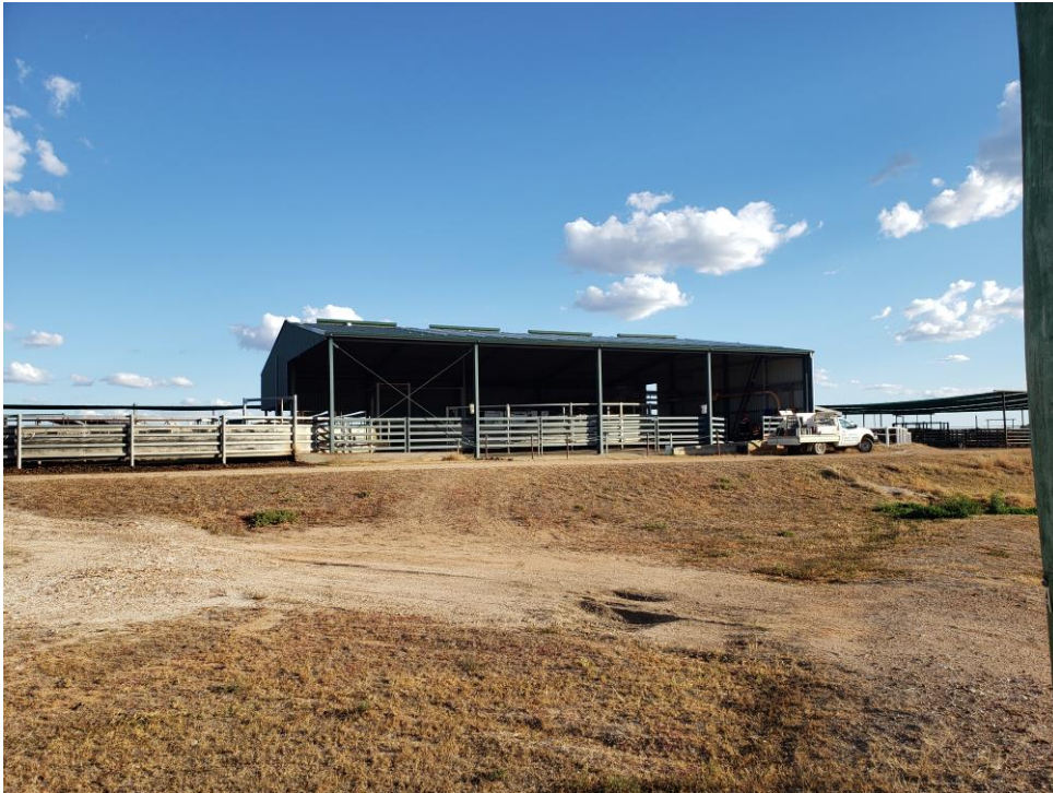
Figure 3: new 29kW p rooftop system under construction during the project period
