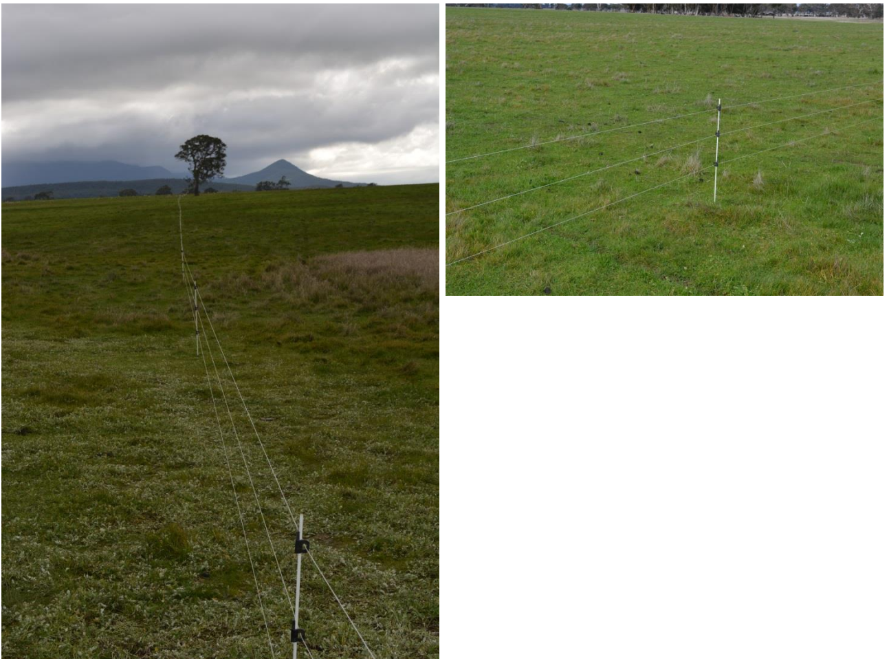
Fig.4 – Fence one after construction and insulated fibreglass tread ins spaced approximately 15m apart
