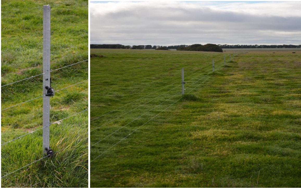
Fig.9 – Design of fence four incorporating four plain wires (2 electrified) and galvanised start posts spaced 15m apart
