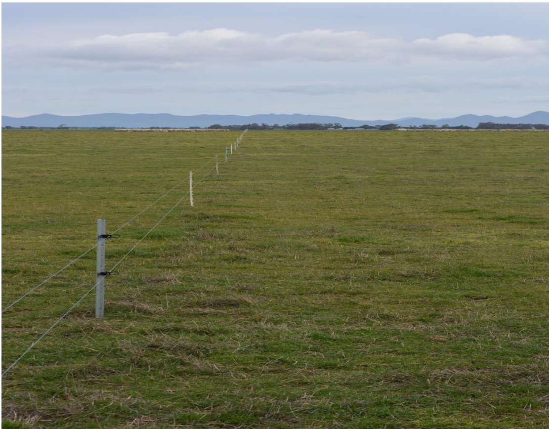
Fig.8 – Fence three after construction
