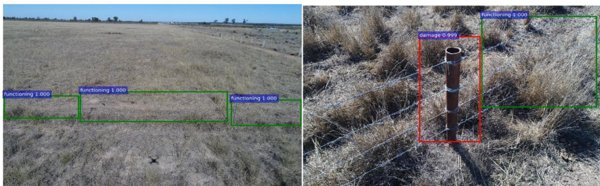
Fig. 44: Type-1 functioning (left), Type-1 damage due to corrosion (right)
