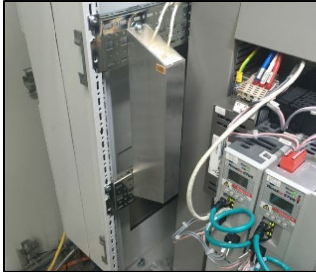
Fig. 25: 400W Shunt resistor that was overheating with the new cycle modifications
