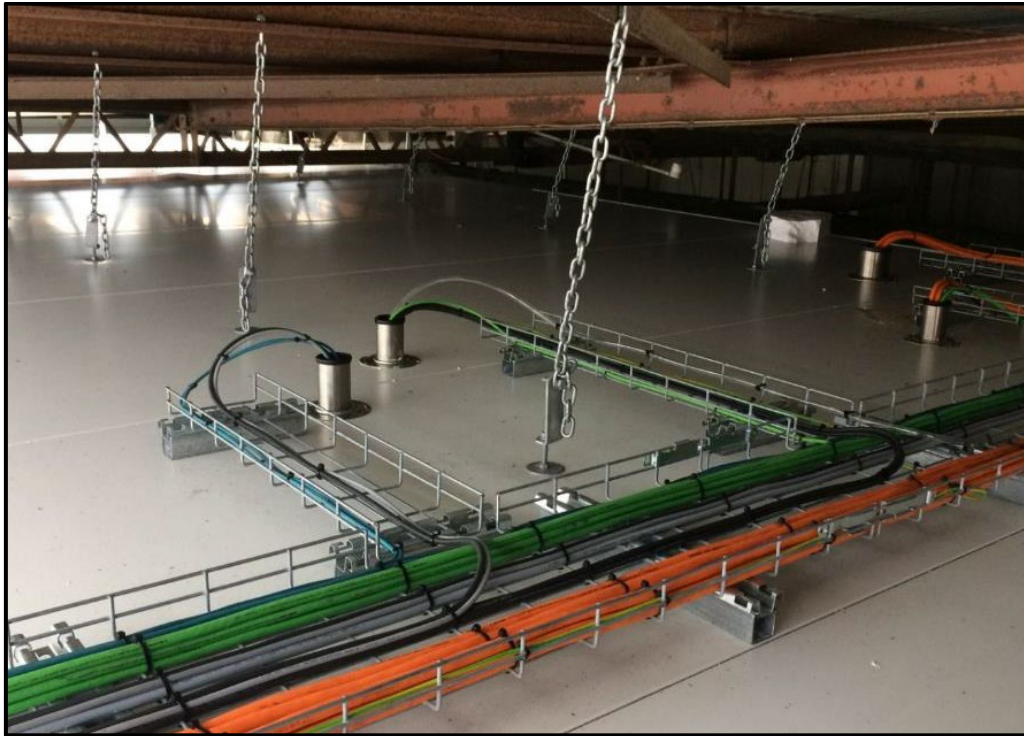
Fig. 12: Overhead Electrical Tray and Duct
