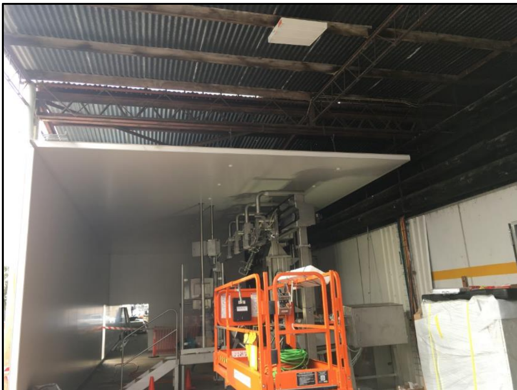
Fig. 10: Ceiling and Wall Constructed Around Primal Tower Components
