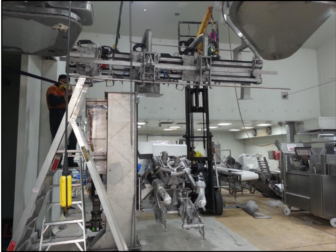
Fig. 11: Overhead transfer being moved into position
