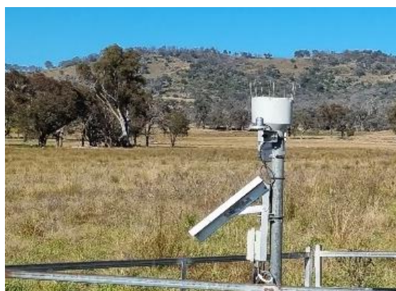
Figure 5: Rain gauge and solar panel installed at Myanbah.
