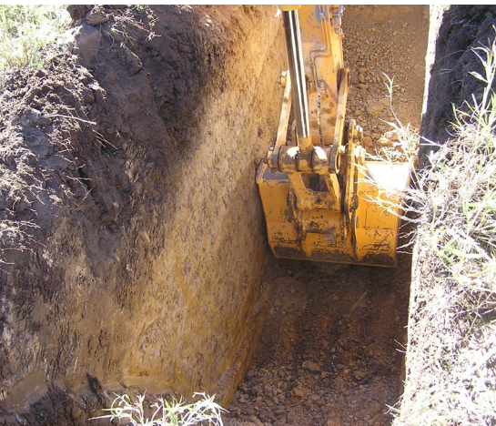
Geotechnical information of the site is gained by excavating test pits, sampling and analysing the engineering properties of the soil material.
