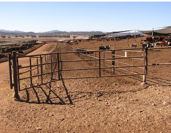
A natural slope of 2–4% allows for drainage and minimal earthworks for site development. Steeper slopes may encourage erosion.
