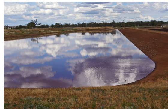
Well-maintained embankment batters with sufficient freeboard
