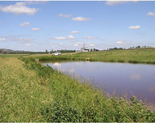
A well-grassed embankment will resist erosion.
