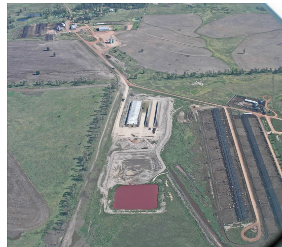
This holding pond was located a sufficient distance away from the closest two rows of production pens to allow for future expansion of the feedlot.
