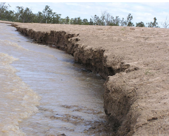
Lack of vegetative cover and a highly dispersive soil allow wave action to erode this internal batter.
