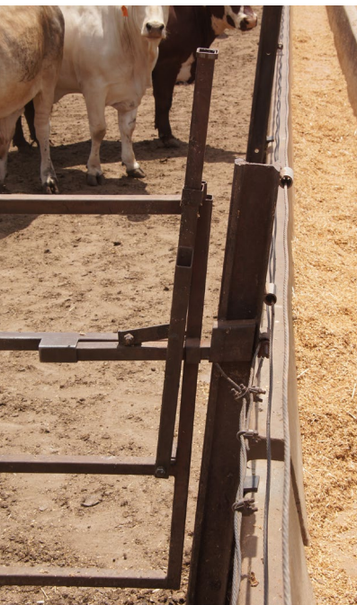
The circular grip on this telescopic pipe latch minimises the risk of pen riders getting snagged. Half circle gate stops prevent cattle damaging the latch when rubbing and allow the gate to be opened in one direction only.
