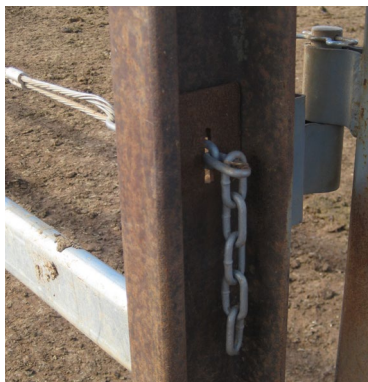
Cable tension is achieved and maintained by locking the cable in the railway line using chain links.
