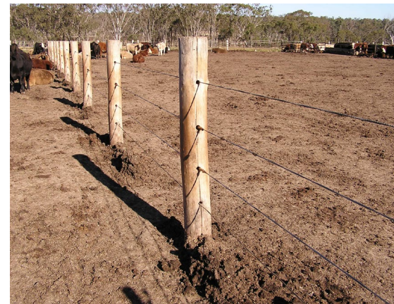
Cables can pass through wooden posts minimising corrosion and cable fraying. This fence line has no top or belly rail.
