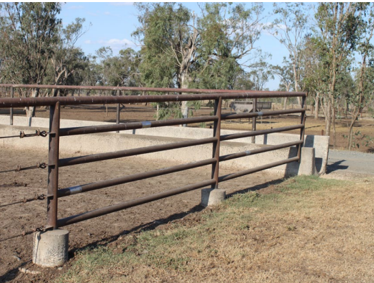
Steel pipe is probably the most common material for fence line posts. Concrete 'post pots' reduce corrosion and also damage by pen cleaning equipment.
