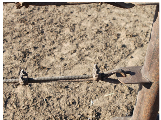
Cable clamps are often used to retain cable tension.
