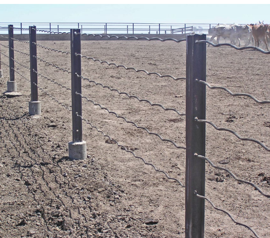
Secondhand or surplus materials from other industries are commonly used e.g. railway line and bore casing.
