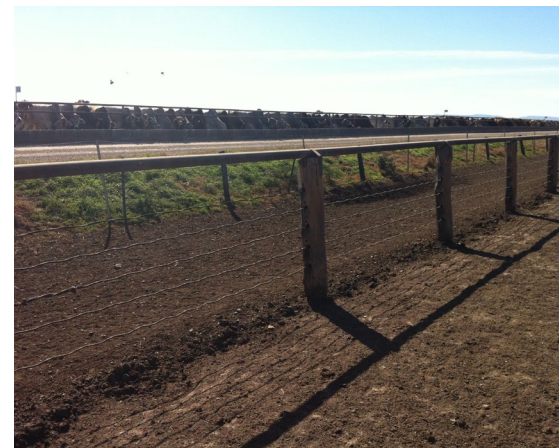
Good quality timber is becoming difficult to source. A steel capping rail will prevent posts without concrete footings from leaning under pressure from cattle.
