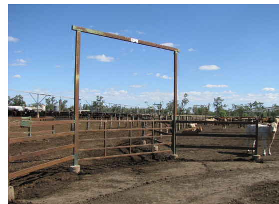
Strainer assemblies across gate openings provide structural stability for both the gateway and cable tension.
