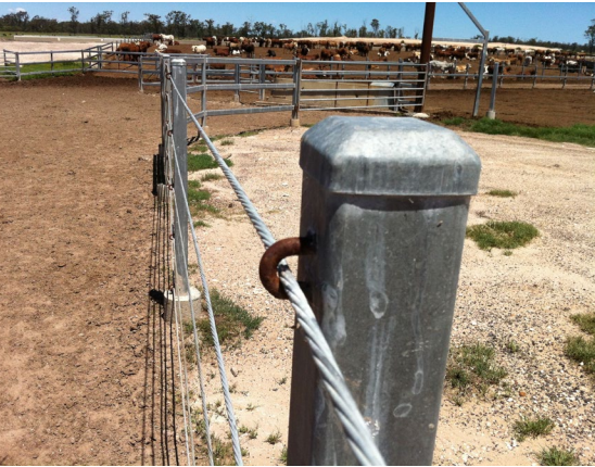
External eyelets hold cables running past steel posts. Hollow posts are capped to exclude water.
