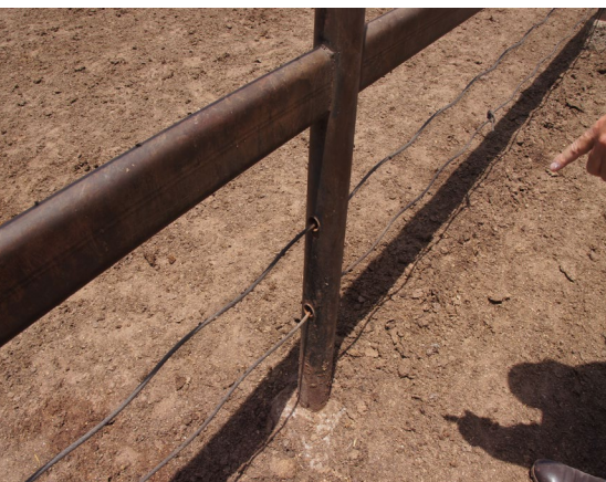
Cables passing through steel fence posts need a steel sleeve to reduce fraying. Sleeves prevent water entering the hollow post but can accumulate moisture which accelerates corrosion of the cable. This is an expensive fabrication technique.
