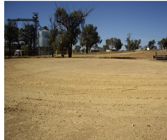
Even grading material on turnaround results in little displacement of coarse material.
