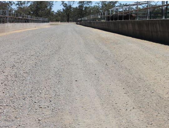
Road constructed from even grading material—well maintained by regular cleaning and grading.
