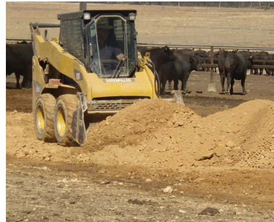
Poorly graded material being used in pen repairs – note the large percentage of fines.
