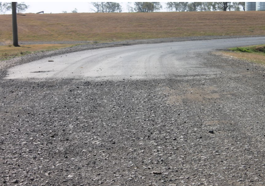
Gravel loss and structural issues are most common on road curves where shear stresses from vehicle loadings are the highest. Bitumen seal on road curves reduces road maintenance but potholes can form easily at the transition with the unsealed section.
