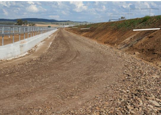
Coarse-graded material used in road construction— larger stones have been graded to the shoulder.
