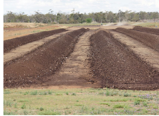
Composting areas also need an impervious base and an even slope of 1–3%.
