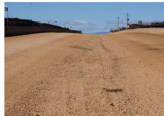
Road cross section – back to back layout with cross-fall to centre of the feed lane and longitudinal fall along the road
