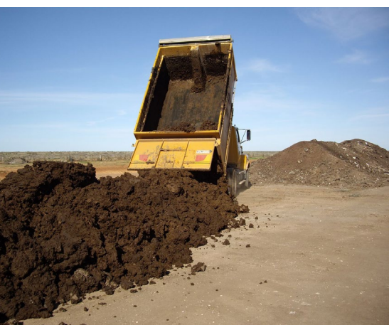
Manure stockpile areas need an impervious base with good site drainage to withstand heavy loads and equipment.
