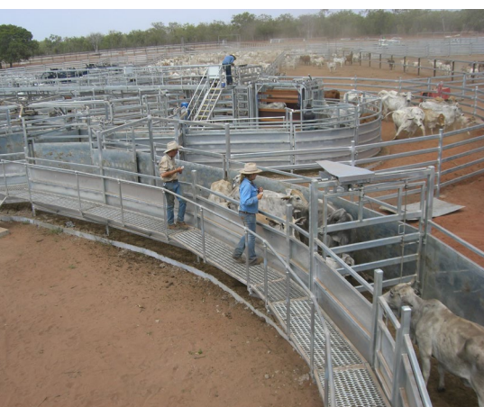
Curved races encourage steady movement of cattle. Operator safety is promoted by external walkways that separate cattle and handlers.
