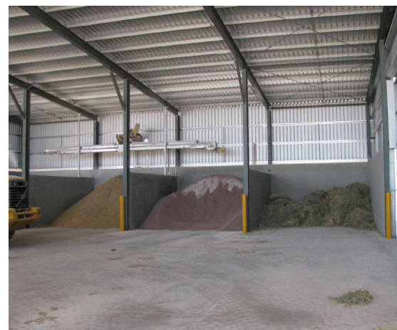
Commodity storage shed with multiple storage bays.
