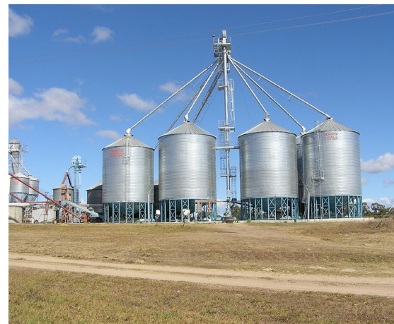
On-site grain storage facility.
