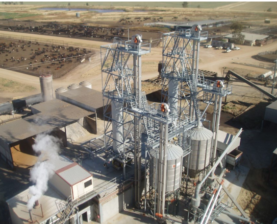
Large feed mill and commodity storage.
