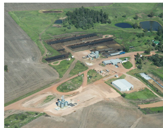
Feedlot undergoing expansion. The old feed preparation and storage area is next to existing pens and a new feed mill is being constructed central to both new and old pens.
