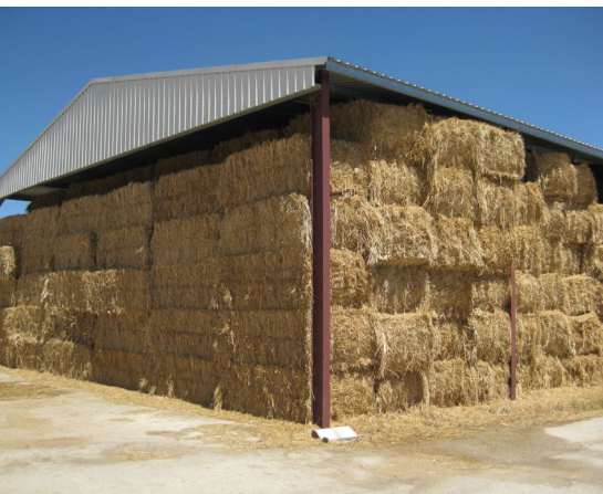
Hay storage in open-sided shed.
