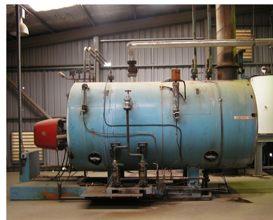
Boiler for the steam-flaking process. Steam generation is the largest single consumer of energy in a feed processing facility.
