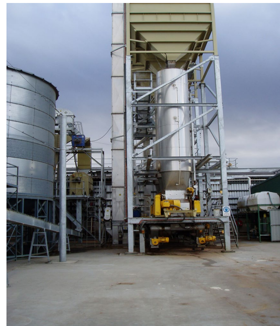
Steam-flaking - grain is transferred to green holding bins above the steam chest. After conditioning in the steam chest, grain enters the flaking mill.
