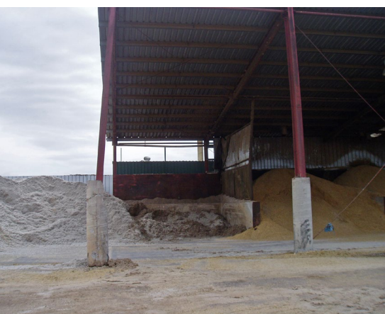
Concrete placed around structural members offers little protection, as the impact is transferred directly to the steel member.
