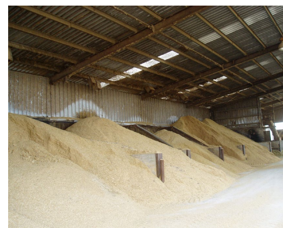
Length and width of individual bays and height of divider walls should be designed to match the volume of material to be stored. Grains with a flatter angle of repose will form flatter piles.
