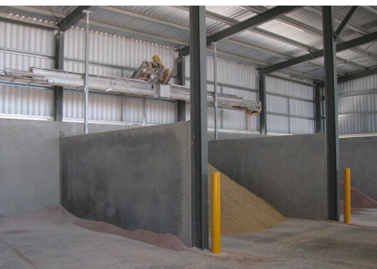
A cross conveyor can transfer grain into one or more bays. Highly visible bollards protect structural members and walls from damage by machinery.
