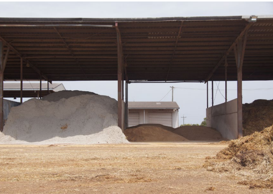
Large push-through bays allow fresh material to be accessible over time.
