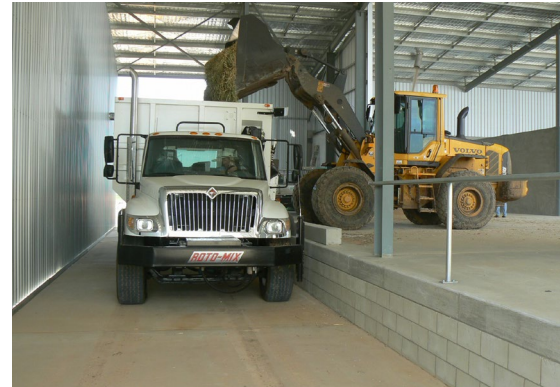
Differing heights between the commodity storage area and the feed vehicle loading bay allow ease of operation and safety.
