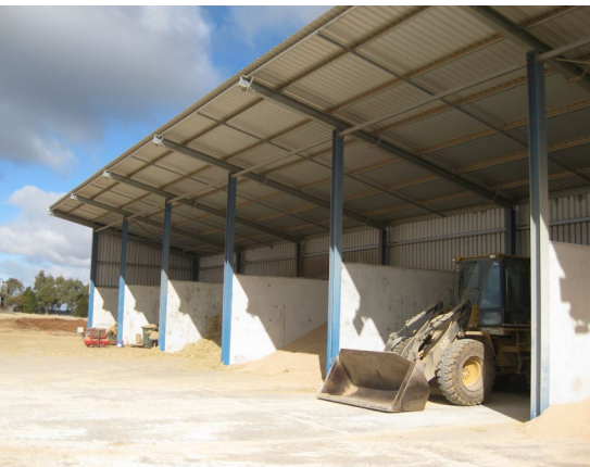
Filling commodity bays by loader can be time consuming and can interrupt loading of feed trucks.
