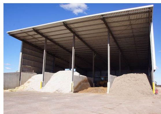
A purpose-built, stand-alone commodity storage shed. The high roof allows direct loading of storage bays from a tipping-trailer truck. A large concrete apron in the front of the bays allows easy vehicle manoeuvring.
