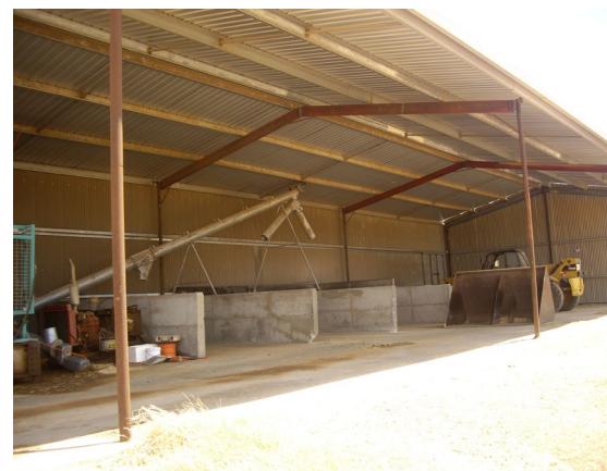
Any storage facility may be adapted to store feed commodities. The side wall from this machinery shed has been removed and storage bays constructed.
