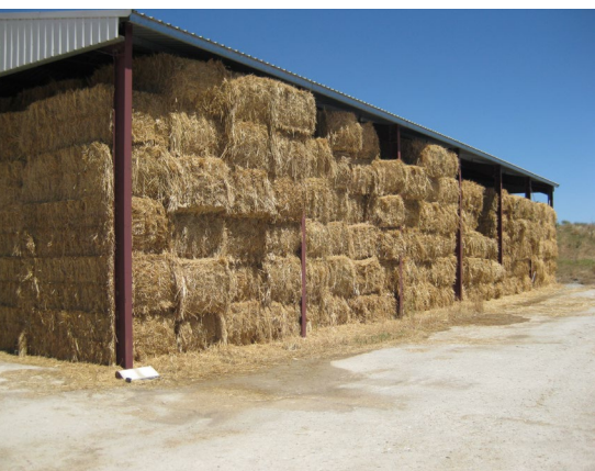
A steel framed, fixed roof open shed. Bales are more likely to be stacked on the stringed side to increase stack stability (as opposed to the unbraced side).
