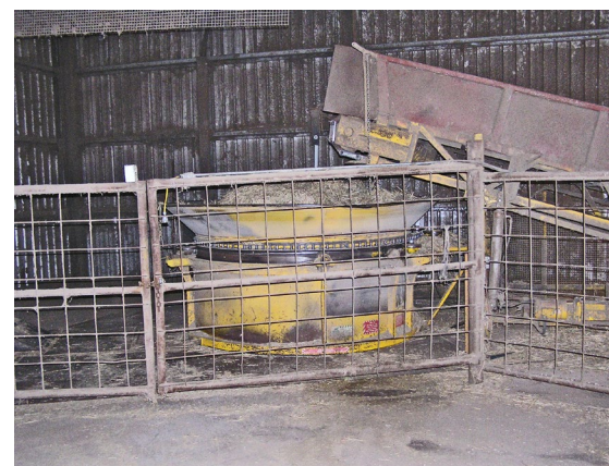
A permanently positioned electric powered tub grinder with the discharge conveyor set below ground level. This arrangement inside the commodity shed presents a greater fire hazard than a portable self contained unit that is easy to access and clean down.
