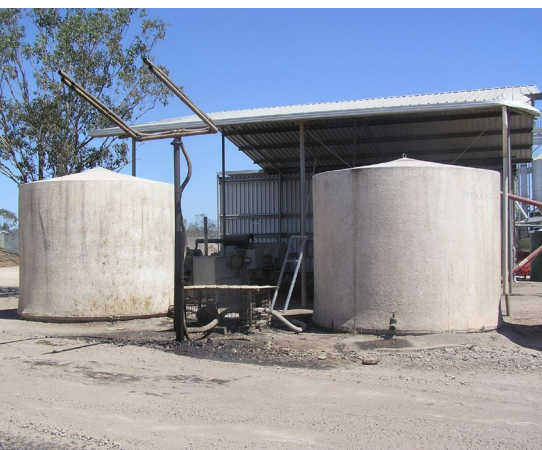
A well-prepared site with a solid foundation for liquid ingredient storage tanks. Flat-bottom concrete tanks are commonly used.
