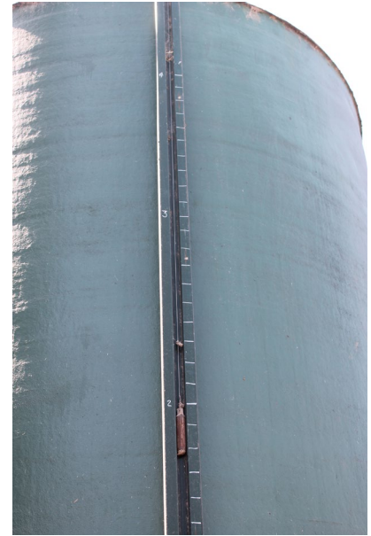
Level indicator fixed to the outside of a storage tank allows inventory levels to be easily checked and recorded.
