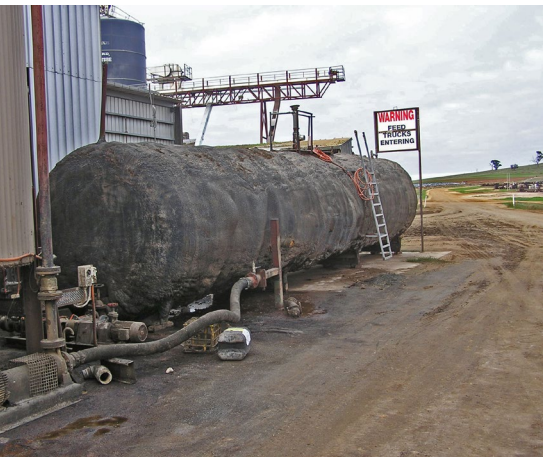
Insulation may be required for those liquids that thicken in low temperatures.
