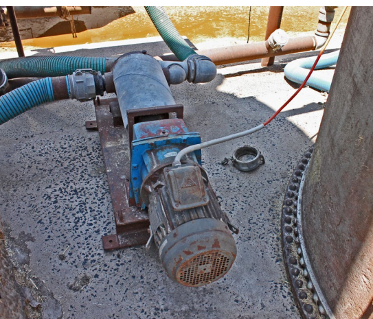
Handling equipment should be of adequate size to deliver the liquid to the delivery point. Larger diameter pipes are required for viscous feedstuffs, such as molasses.
