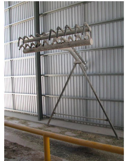
Liquid feed-out station. Storage tanks and pumping equipment are located on the outside of commodity shed wall with a delivery pipe through the wall.
