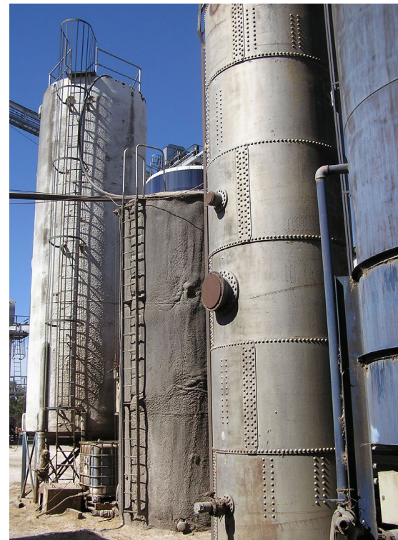
A bank of conical and flat-bottom steel tanks. Filling point is easily accessible at ground level, or at the base of conical tanks. Note there is insulation on some tanks to keep liquid warm and reduce viscosity.
