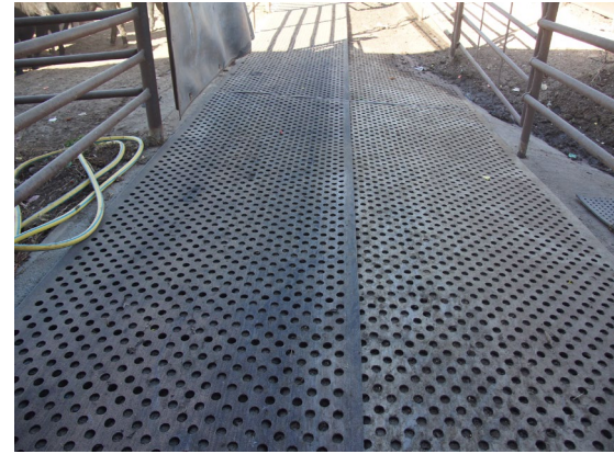
Rubber soft-flooring in handling areas.
