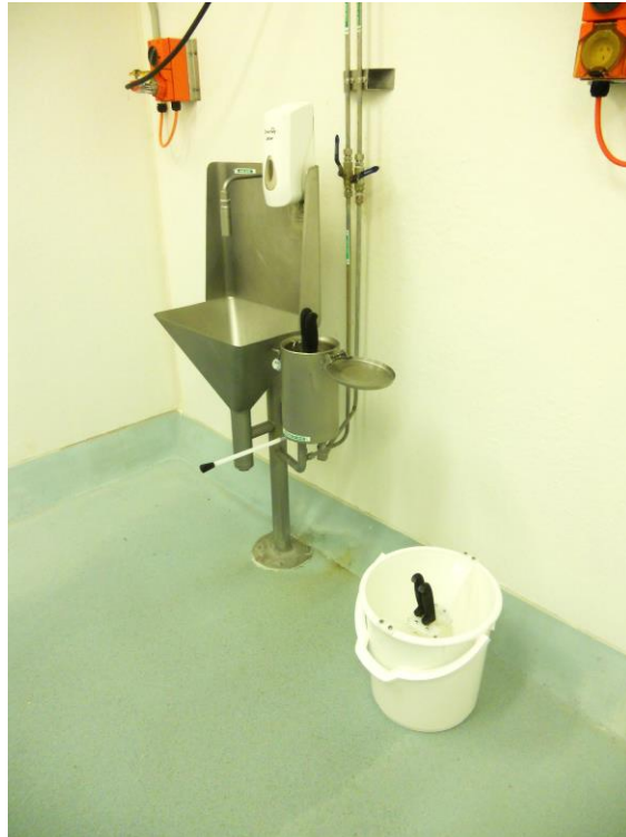
Figure 1. Trial knife set up, hot water sterilisation set up and bottom right is the chemical sterilisation knife holder
